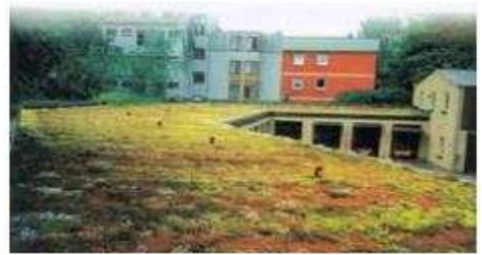
Fig. 1: An extensive roof covers the garage providing an aesthetically pleasing view for the building occupants
